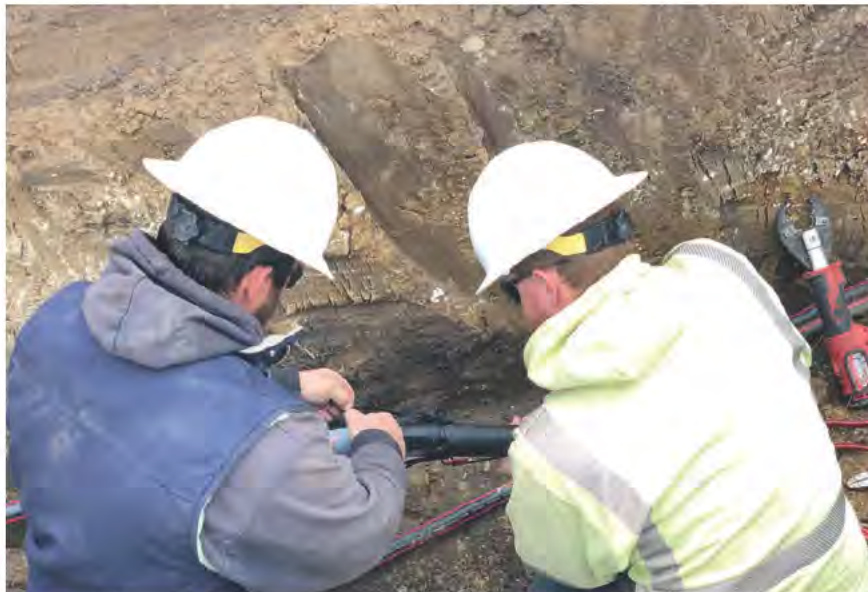
Linemen Tim [redacted] and Chandler [redacted] work on underground installation southwest of Epiphany. The new underground line will help improve reliability in the area.
