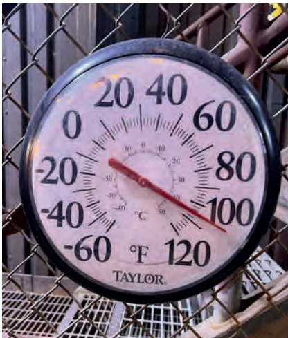
Temperatures reach more than 100 degrees at the top of the Antelope Valley Station boiler.
