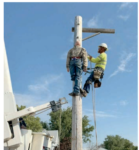
Mitchell Area Foreman Tony [redacted] performs pole top rescue training.
