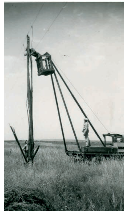
Linemen placing poles in the early days at Moreau-Grand Electric.
