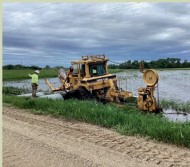
Larson Digging didn't let a little water stop them from plowing in new underground for members south of Mount Vernon in June.
