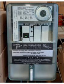
This is an example of a load management receiver. It is required for certain rates and rebates on water heaters, air conditioners and irrigation systems.
