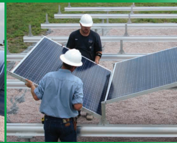
4) Install the panels at an angle, and attach to the previously set braces. Photo: Ryan Bigge & Rodney Weber
