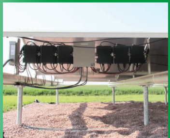
7) Set the redundant inverter bus, which holds the inverter units and is wired to the panels
