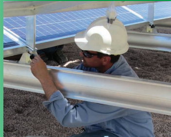
5) After setting all the panels, each is tightened in place and a keeper plug is clipped on. Photo: Daren Hoffer
