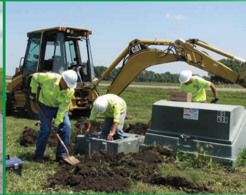
2) Install the transformer & dig the transformer basement. Photo: Tim Harrington, Dustin Weier, & Cody Riggs
