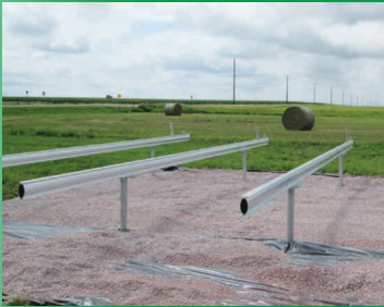
1) After preparing the area, crews anchored the poles and attached the rails that the project would set on.
