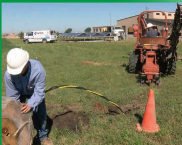
8) Trench underground cable from the solar project out to the transformer. Photo: Daren Hoffer & Kevin Johnson
