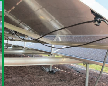
6) Wire each individual panel underneath, which will eventually be connected to the inverter units.
