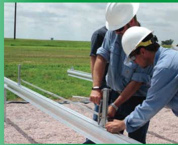
3) Set and space the braces that will hold the panels. Photo: Rodney Weber & Daren Hoffer
