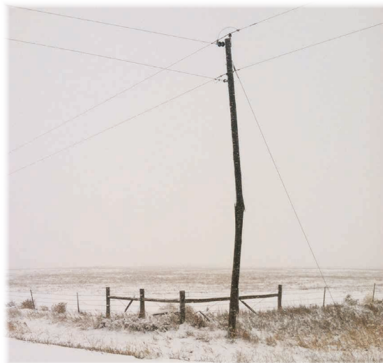
This pole was struck by a car that drove off the road during the winter conditions. These repairs can be costly for the cooperative.
