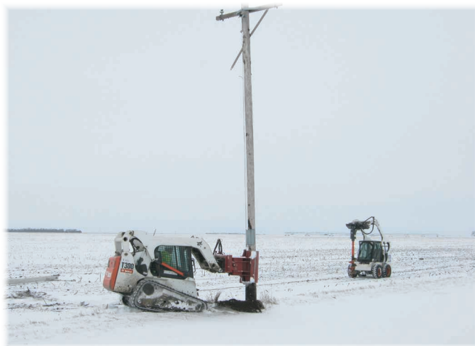
Crews retiring overhead line that had been converted to underground line earlier in the season.
