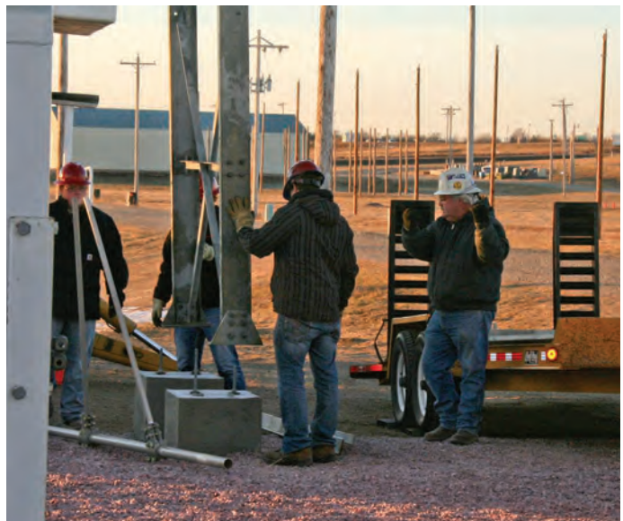
Above & Below: Instructor Jerry Ehlke supervising the construction of a steel structure at the substation facility
